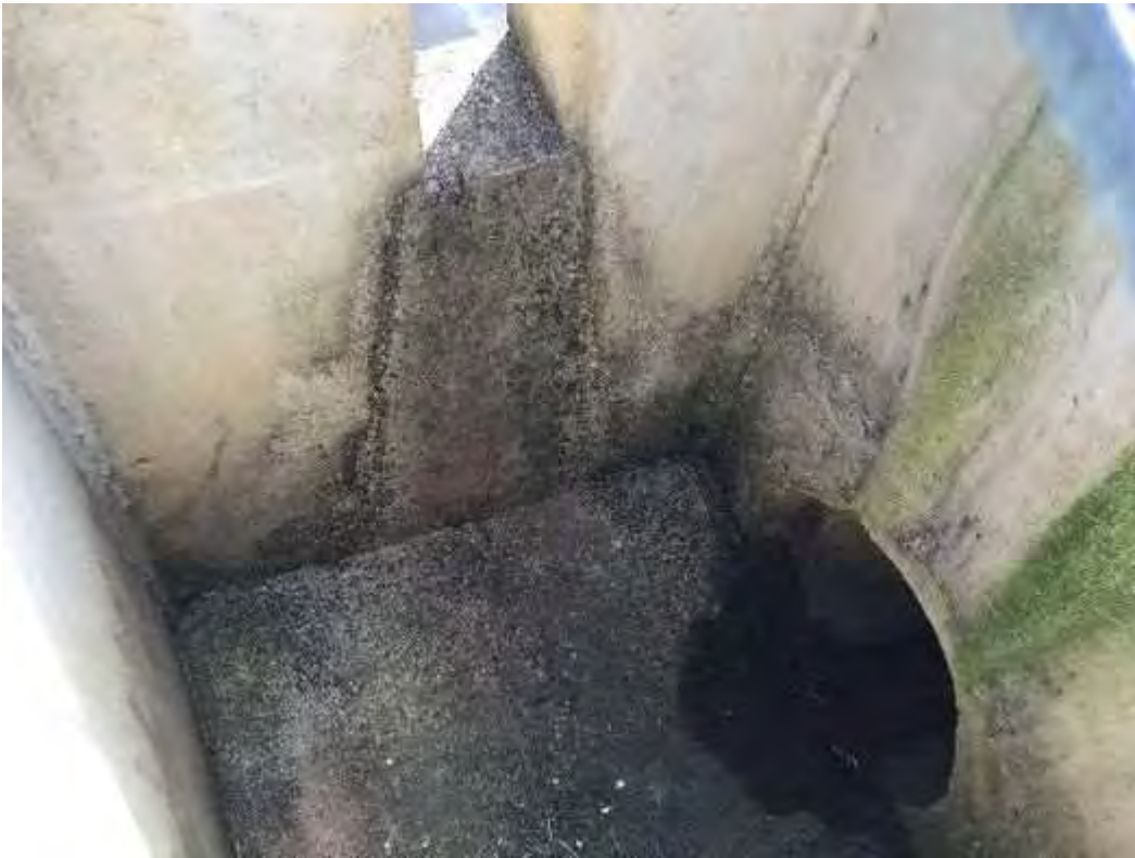
Control Structure (interior)
