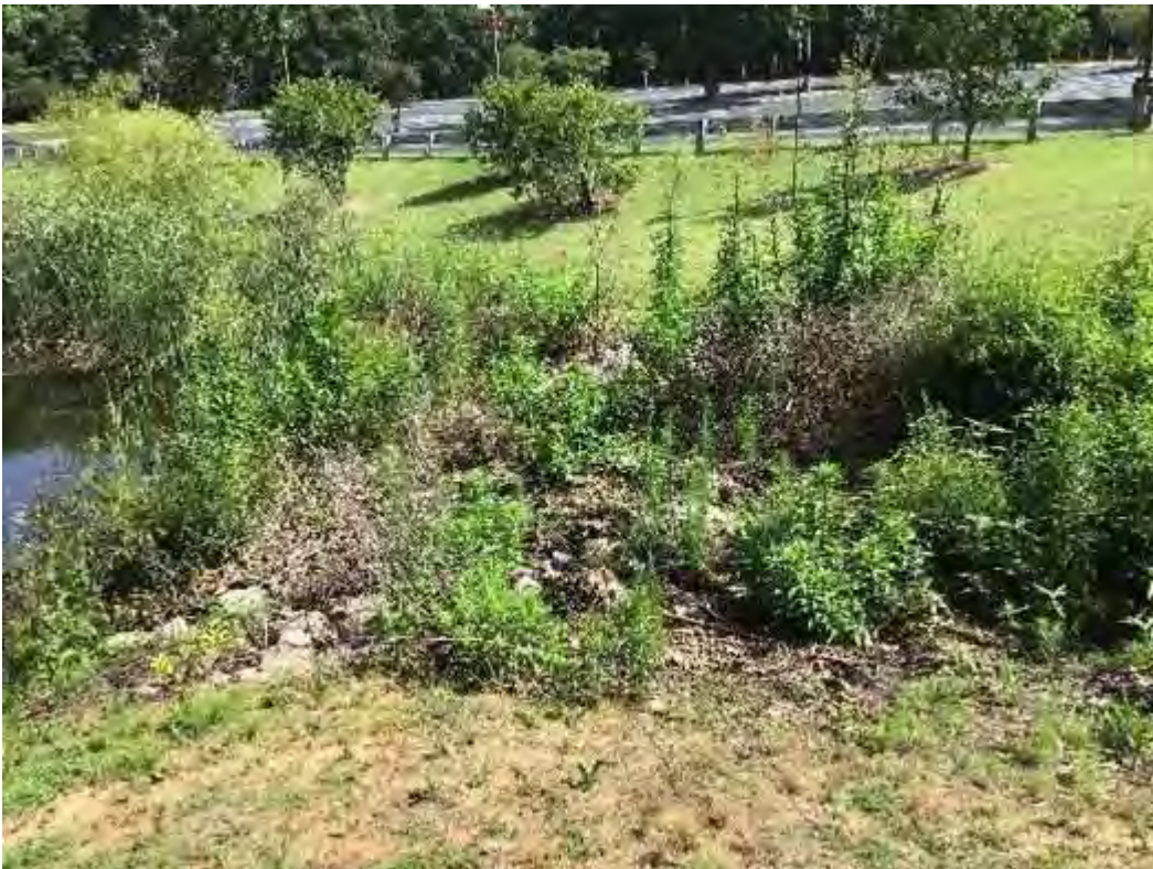
Forebay Weir (note overgrown vegetation)
