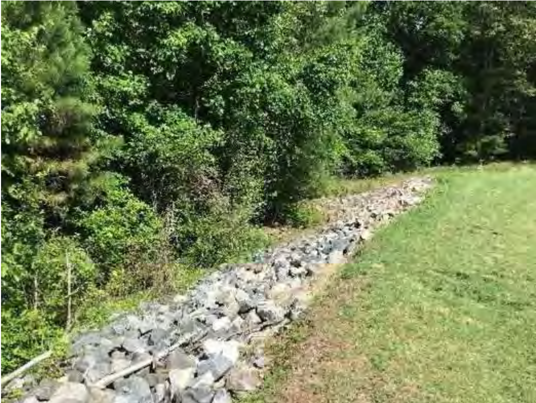
Downstream Embankment Slope
