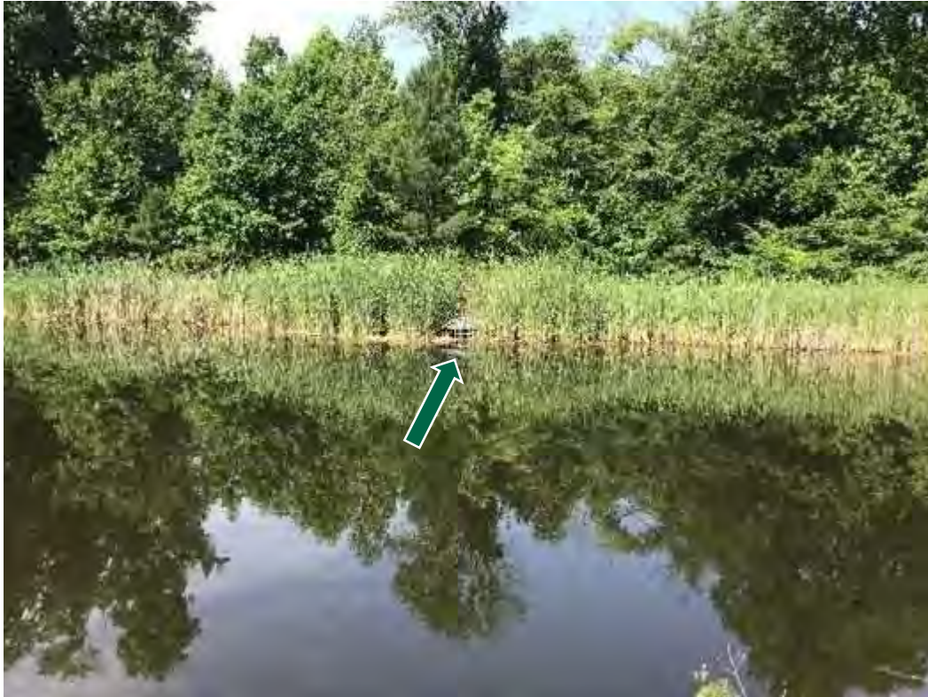
Control Structure (arrow)
