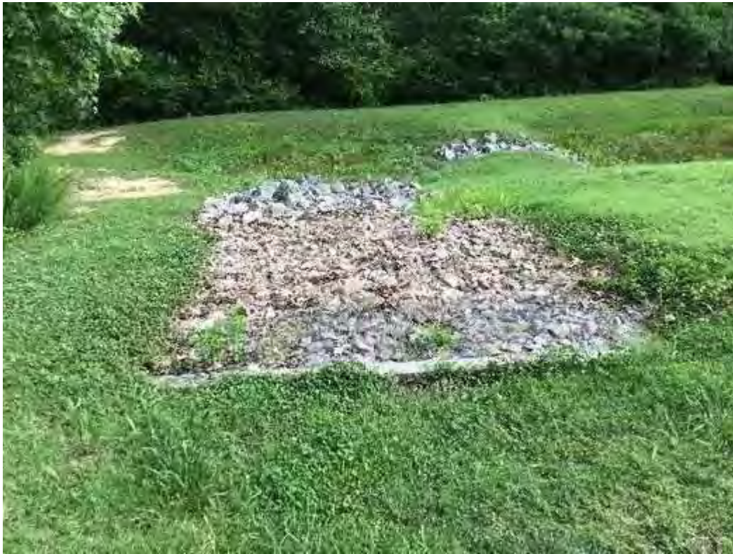
Level Spreader Inlet (into forebay)
