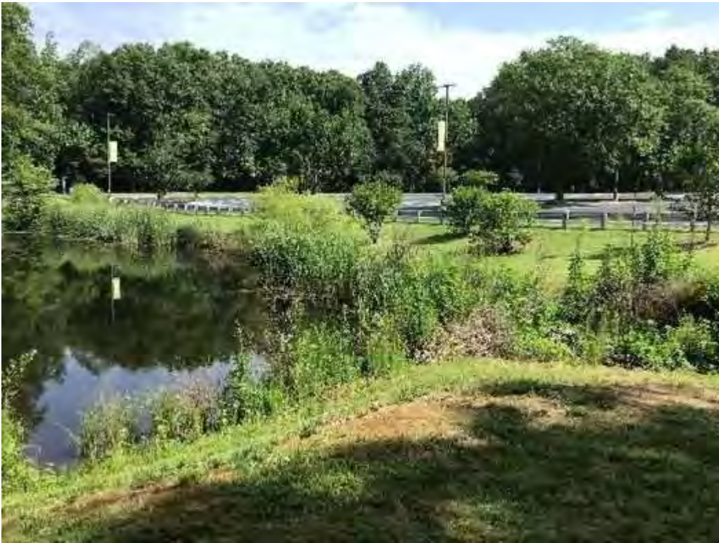
Forebay Weir Overflow
