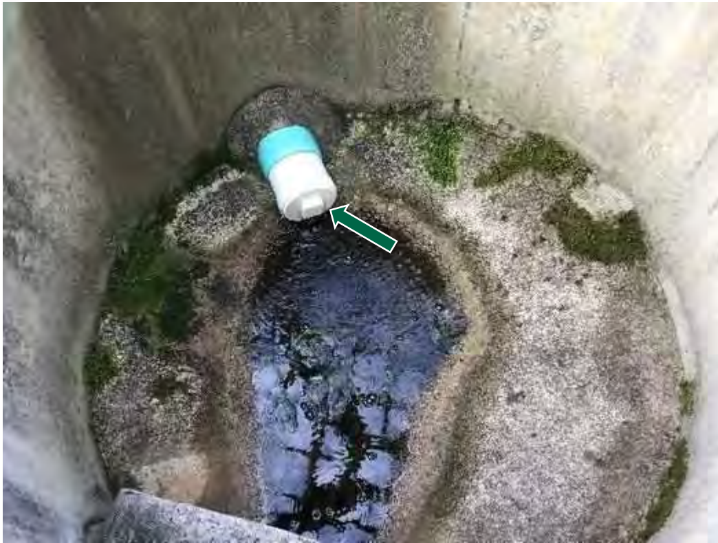
Control Structure Interior (note orifice plug, arrow)
