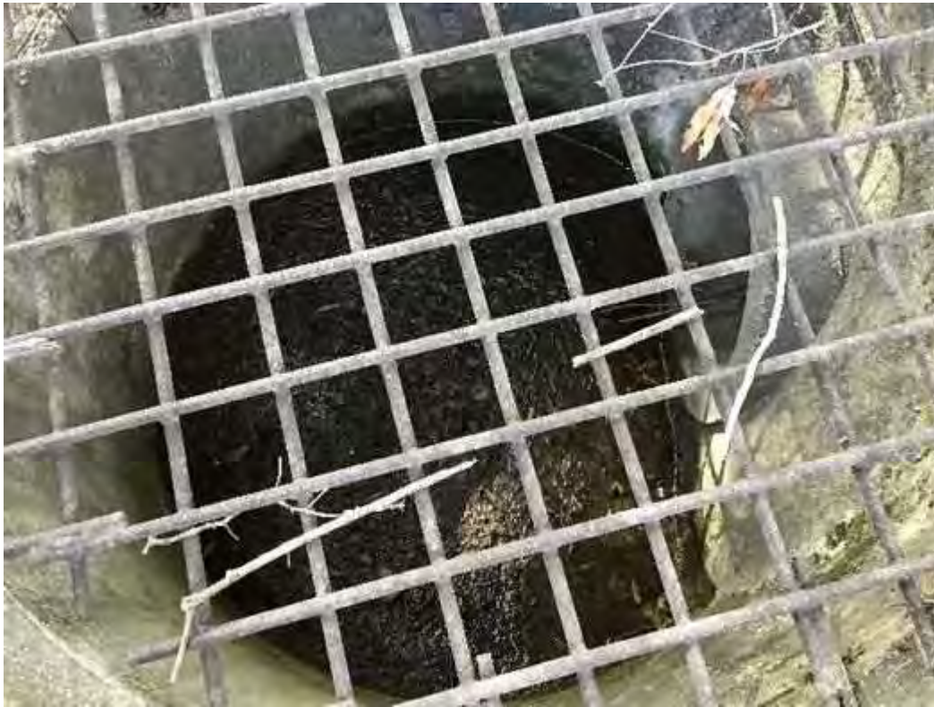
Control Structure Interior
