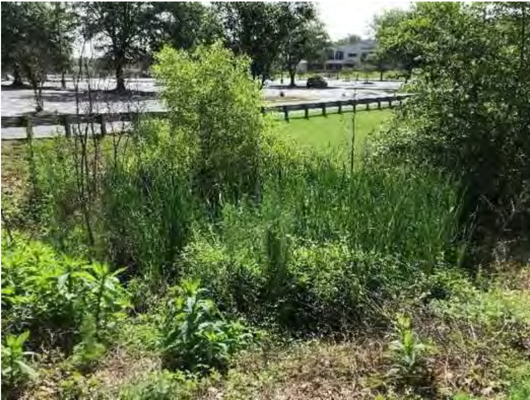
North Inlet (note overgrown vegetation and trees)
