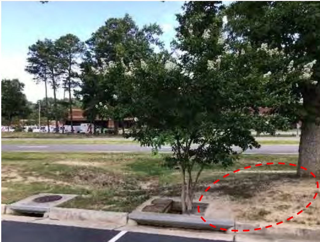
Note Unstabilized Area (circled) Upgradient of BMP
