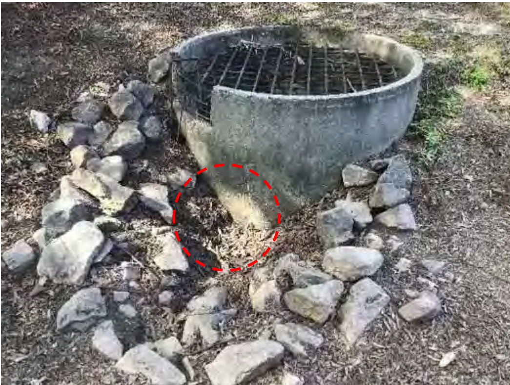
Control Structure (note low-flow orifice, circled)
