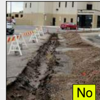
Trench in Asphalt
